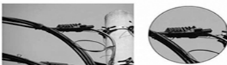
Gambar 3.10 Strain Clamp
